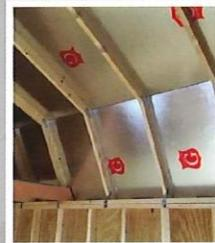
Roof sheathing designed to reflect up to 97% of the sun's radiant heat - keeping it from being absorbed into the building. That means you can maintain indoor comfort while lowering peak temperatures up to 30°F. This high-quality roof sheathing combined with Graceland's patented "Soffit Ventilation System" creates the "coolest" buildings in the market!
